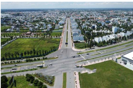
Loc Giang Industrial Park Ready to be put into business from 2026
