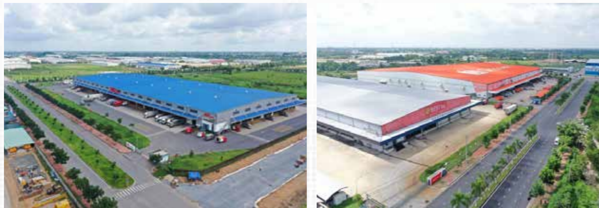
Factories under construction in Tan Phu Trung IP
