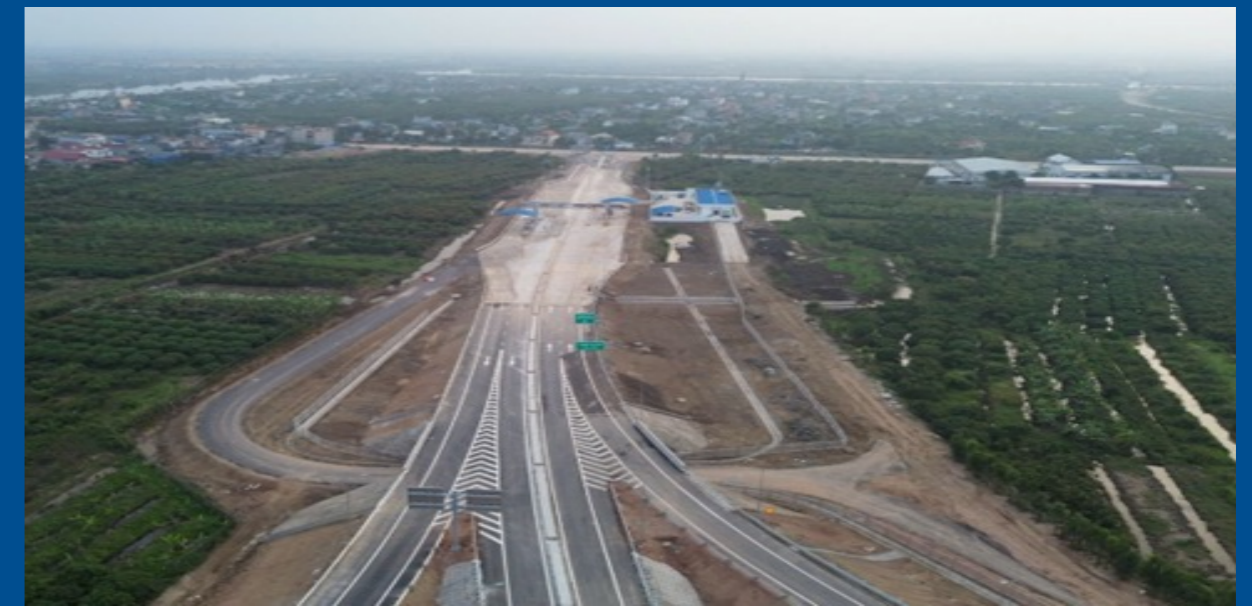
The interchange connecting Provincial Road 390 with the Hanoi – Hai Phong Expressway was officially opened to traffic on February 12, 2026
