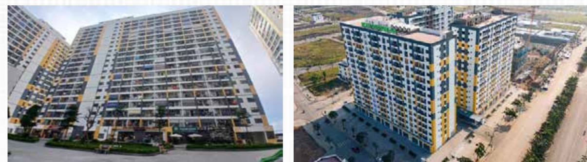
Nenh Town SH Project and Trang Due SH Project
