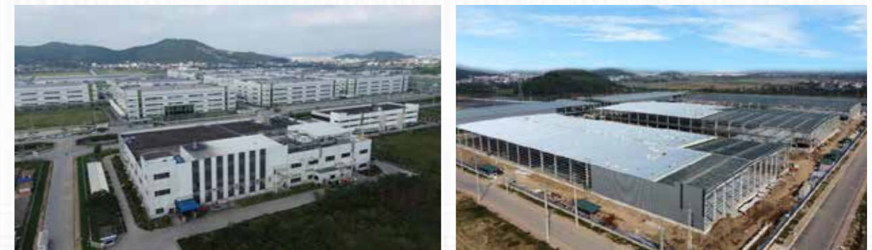
Factories under construction in Nam Son Hap Linh IP
